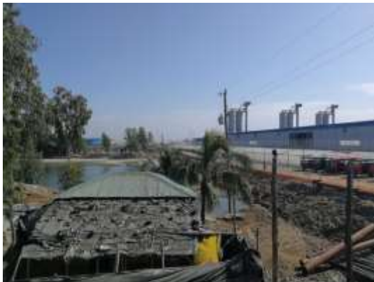
Figure 1. Conditions by the northwest gate. The project site is on the right-hand side.
