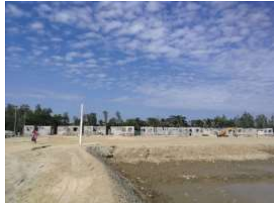
Figure 2. Alternative housing for relocated residents during construction.
