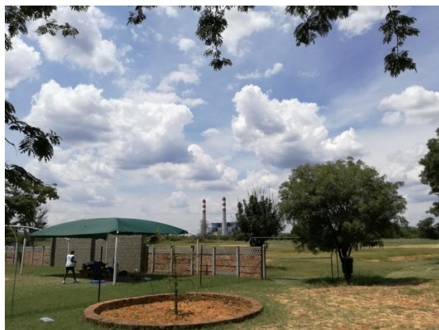
The Elementary School monitoring station
