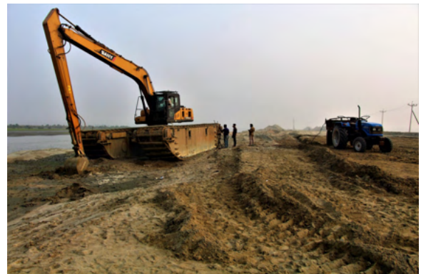
Figure 5. Filling up of the Kohelia river due to the access road construction.
