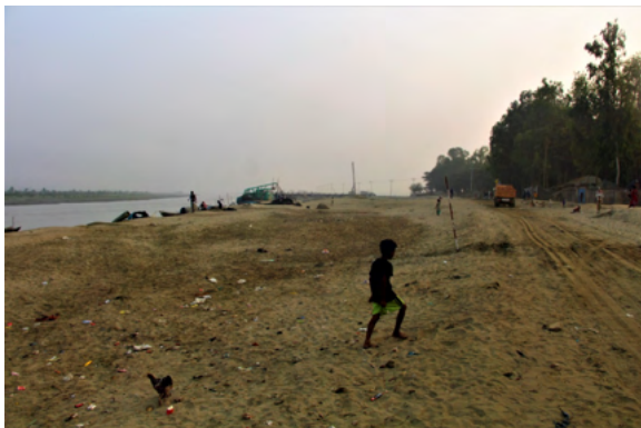
Figure 4. Access road construction along the Kohelia river.
